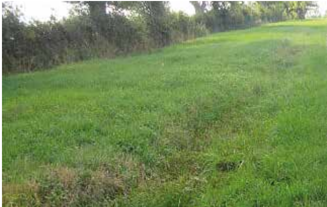
Swale to divert and hold surface runoff © Eden Rivers Trust
