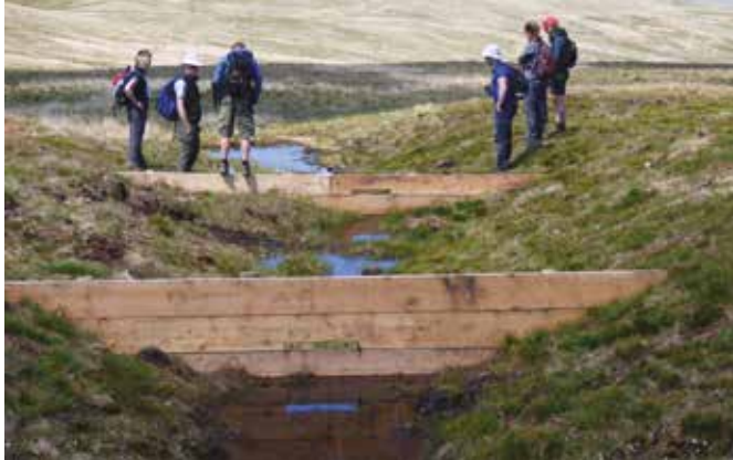
Gully blocking with leaky bunds on Tebay Common. © Cumbria Wildlife Trust.
