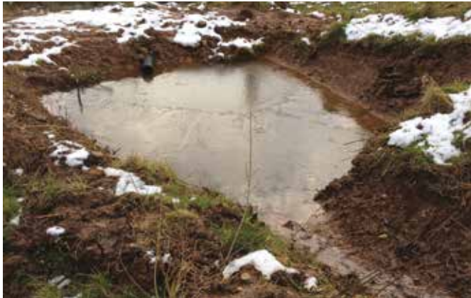
Sediment trap filtering runoff from a farm track before discharging into a stream on River Leven, North Yorkshire. Image © Yorkshire Dales Rivers Trust, with thanks to Tees Rivers Trust.
