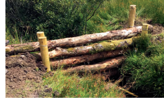
In-channel barriers © YDRT
