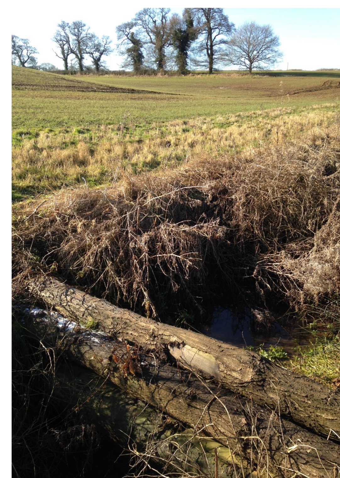
Semi-permeable dam in the Eye Brook catchment (source: Water Friendly Farming Project)
