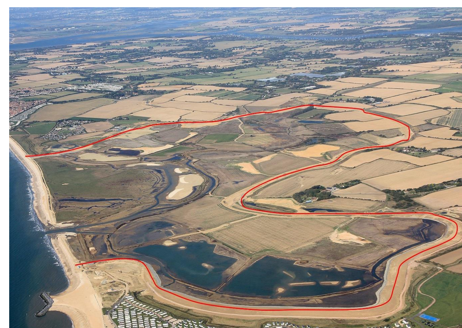
Medmerry managed coastal realignment site, 10 October 2013 (source: Environment Agency and John Akerman ABPmer)
