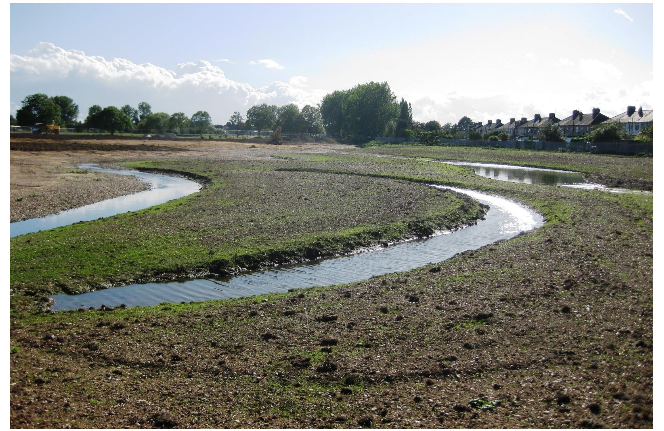
Mayes Brook river floodplain restoration post-construction (source: Environment Agency)
