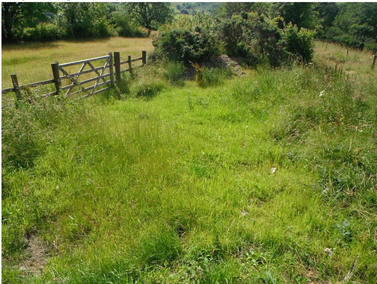
Photo 1: Downstream breach, Low Stranger Farm (source: West Cumbria Rivers Trust)
