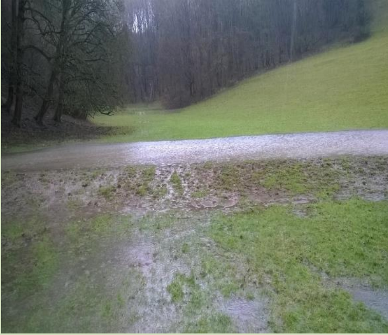
Photo 5: Earth bund retaining water during storm event, December 2015 (source: Chris Uttley, Stroud District Council)
