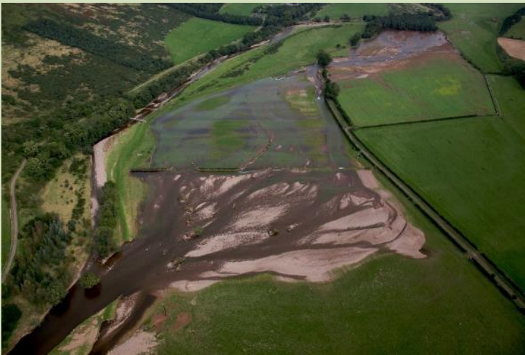
Photo 3: An avulsion on the River Glen (downstream continuation of the Bowmont in Northumberland) caused by the September 2008 flood event. It is thought this happened in part due to excessive sediment supply from the Bowmont catchment.
