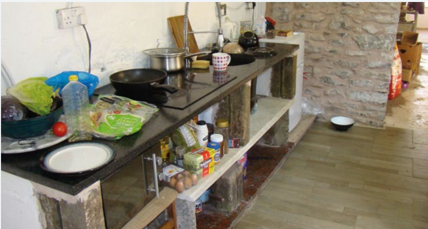
Figure 4 Granite topped kitchen shelving, with marble shelves and sandstone window mullions as a framework – some of the materials were found by the river, having been dumped there 18 months earlier!
