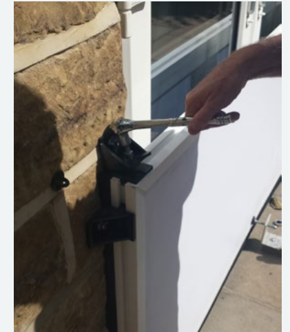
Figure 10 Fitting new (taller but light-weight) barriers
