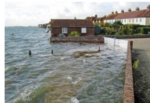
Figure 1 Flood barrier in action
