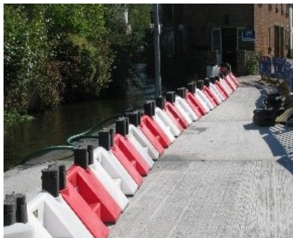
Figure 1 Temporary flood barrier deployed during trials in Wilton
