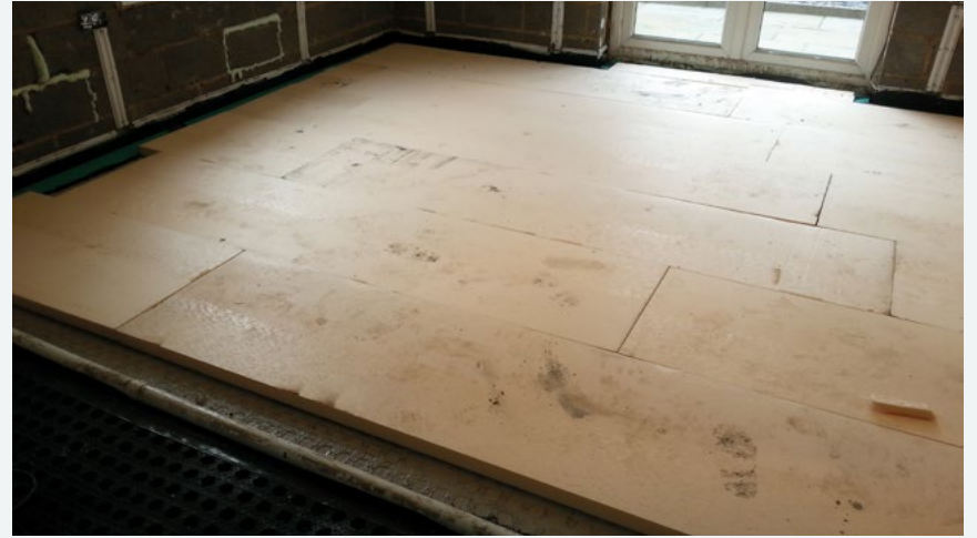
Figure 6 Closed cell (waterproof) insulation on the floor
