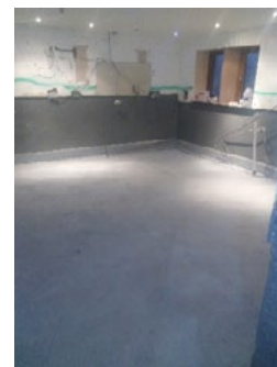
Figure 1 Barn kitchen during work
