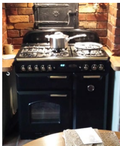
Figure 3 Range in tanked alcove has its own flood barrier
