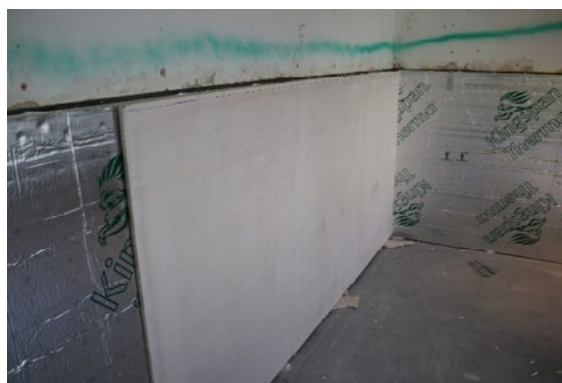
Figure 3 Detail of 'Sandwich' construction for lower walls during work
