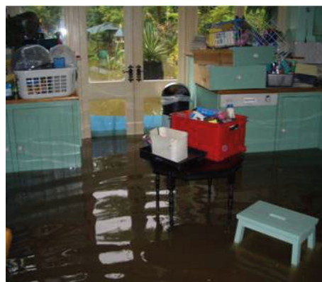
Figure 1 Kitchen during the flood
