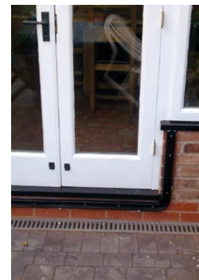
Figure 1 Non-standard doorway with unobtrusive barrier fittings
