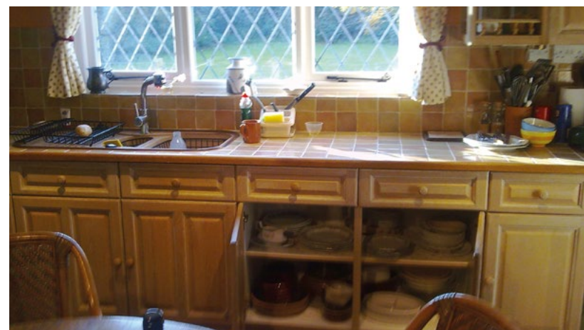
Figure 4 Fitted kitchen with plastic carcasses and removable doors
