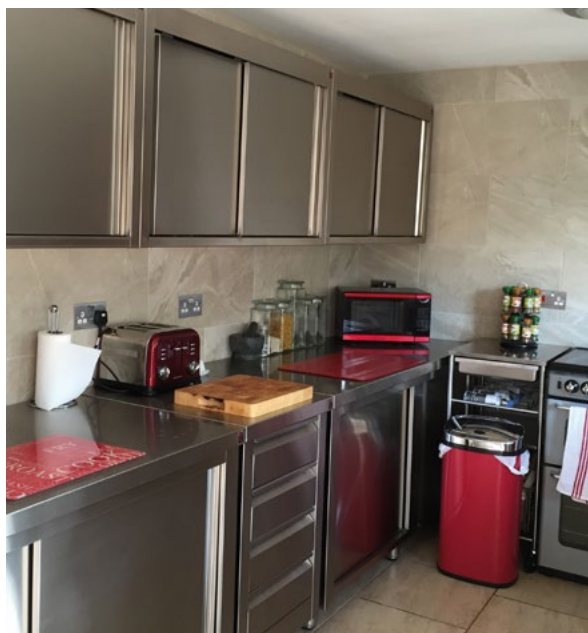
Figure 4 Free-standing stainless steel kitchen with free-standing appliances, which can therefore be moved to safety. The walls are tiled from floor to ceiling, using water-resistant cement and grout; internal door re-hung with hinges allowing it to be lifted off and moved upstairs.
