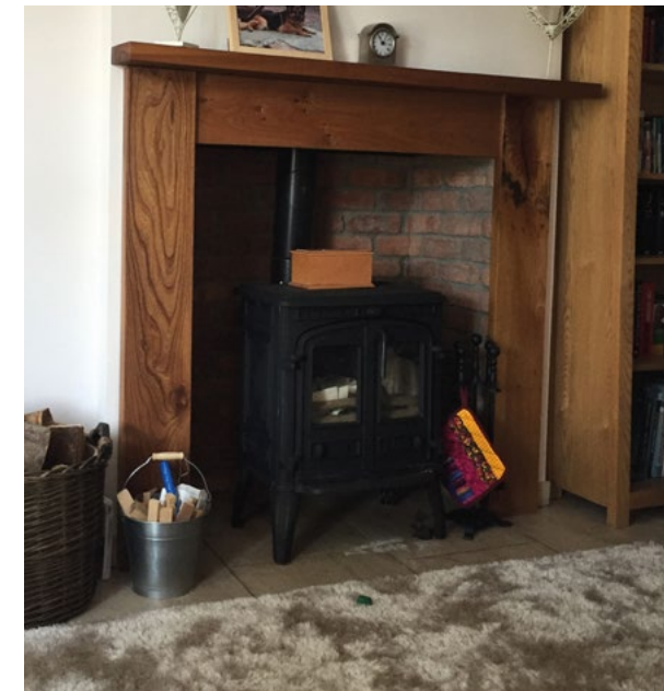
Figure 3 The fireplace surround is also made from hardwood, and has successfully survived a flood
