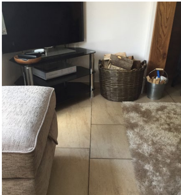
Figure 1 The ground floor is tiled throughout, using water resistant cement and grout – it can be hosed down and disinfected after a flood
