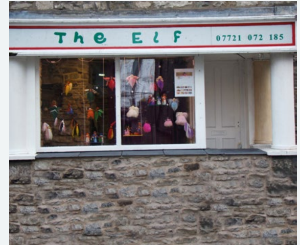
Figure 3 Shop front, with new flood wall to deflect bow waves' caused by passing vehicles
