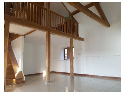
Figure 4 Completed walls Walls sealed with Polyurea (donated by www.adlerandallan.co.uk ) then closed cell insulation applied (by www.kingspan.com ) and finished with Dragonboard (donated by www.dragonboard.co.uk )
