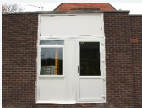
Figure 3 Flood resistant side door donated by www.floodsmartsystems.co.uk
