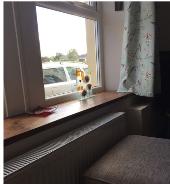
Figure 2 The window sills are made of hardwood (instead of the usual easily-damaged softwood)
