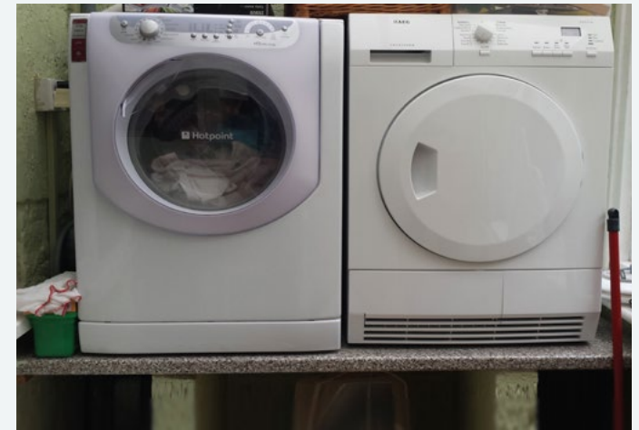
Figure 10 Raised appliances in utility room
