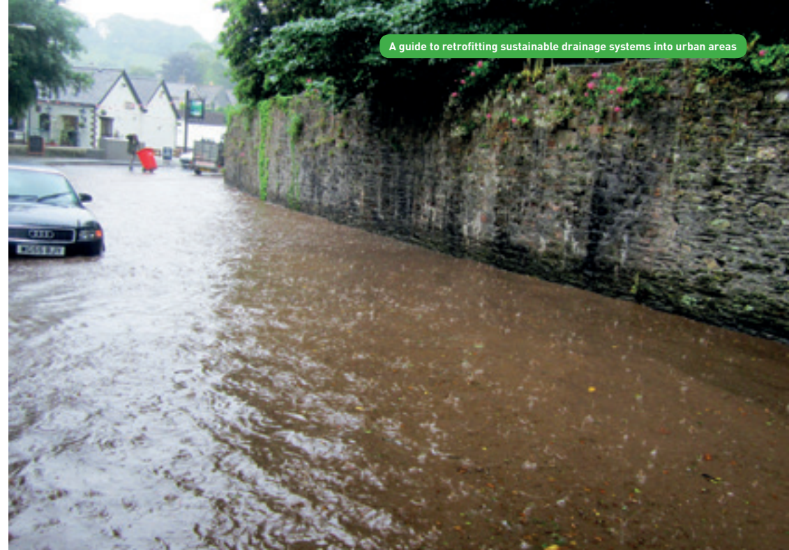
Flooding in Plymouth
