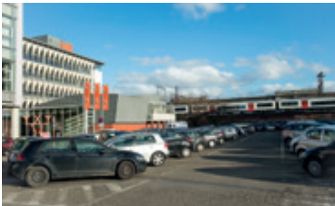
Prior to work commencing
