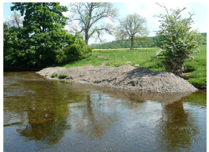
Figure 5: Dredging of the River Lowther
