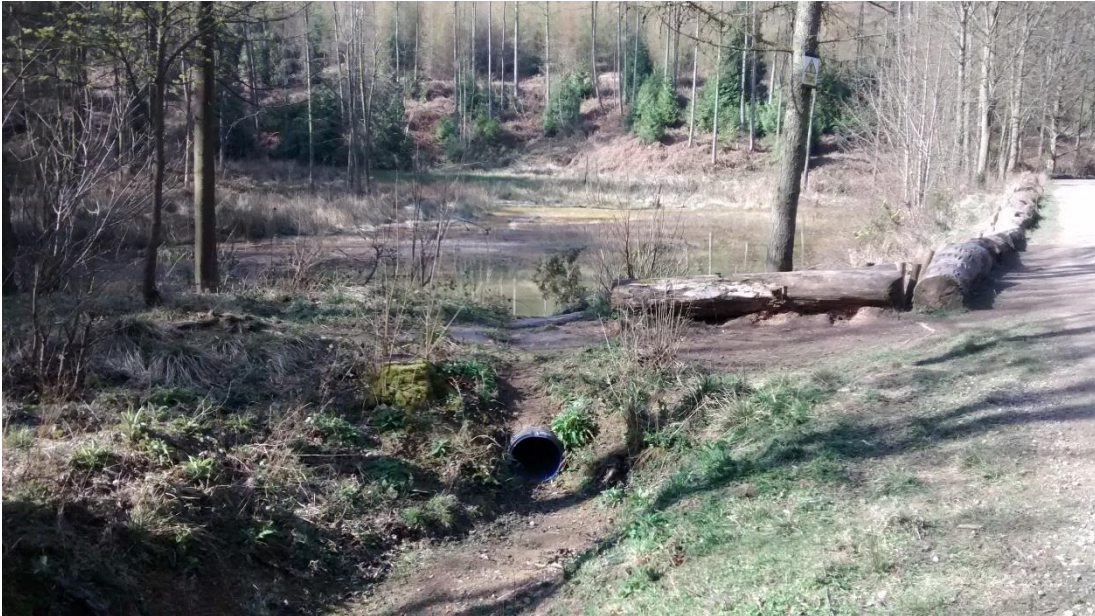
Photo 1: A dam that will be refurbished and made greener as part of the scheme (source: Environment Agency)
