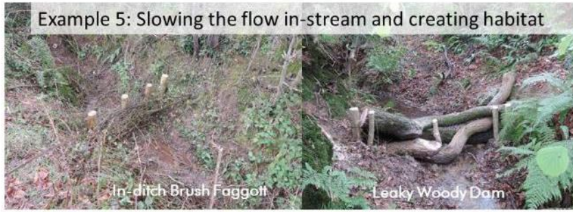
Photo 1: Examples of completed Hills to Levels work
