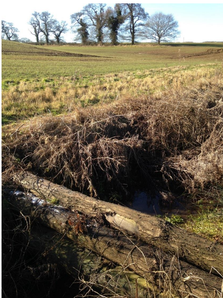
Photo 1: Semi-permeable dam in the Eye Brook catchment (source: Water Friendly Farming Project)
