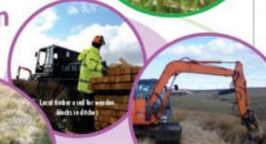
Restoration on Broombe using special tracked diggers with very low ground pressure.
