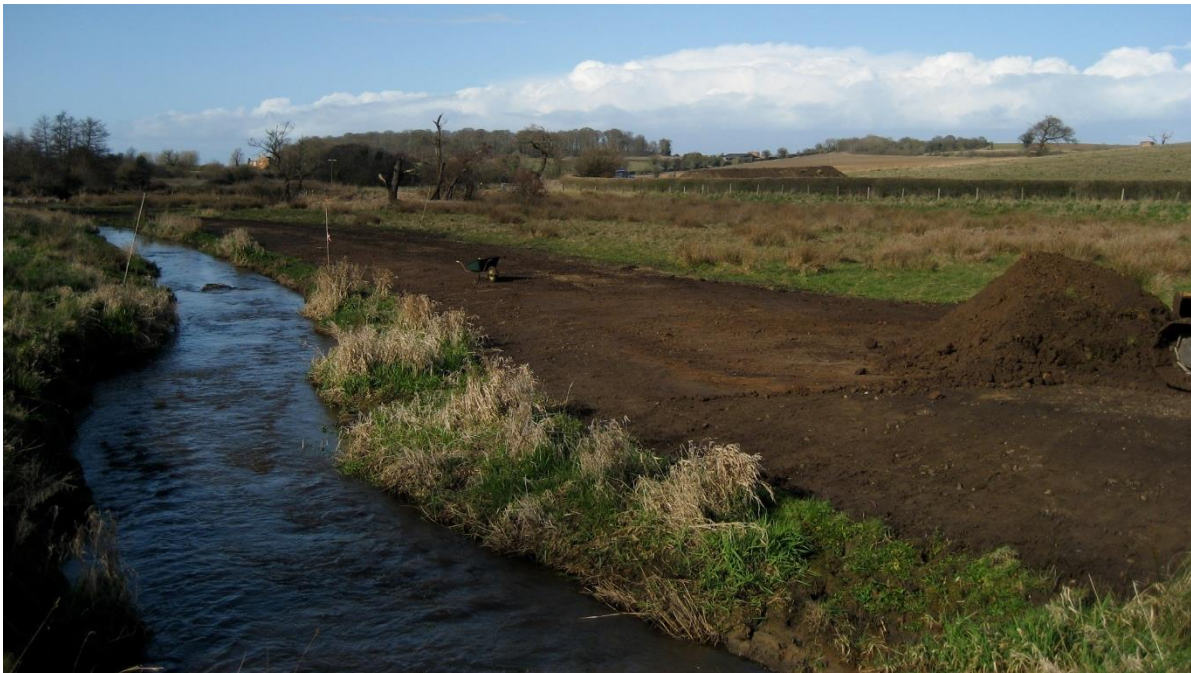
Photo 1: Embankment removal work in progress, 2009 (source: Clilverd 2016)
